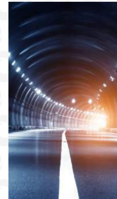
BORIVALI-THANE UNDERGROUND SGNP TUNNEL
